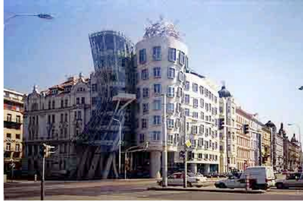
Fig. 6: The corner of the National-Nederlanden Building
